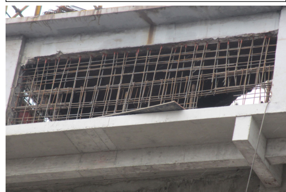
Fig. 1: Retrofitting of Structure using Shear Wall
