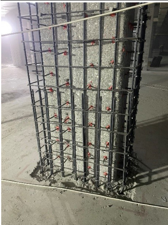
Fig. 2: Strengthening of structures using concrete jacketing
